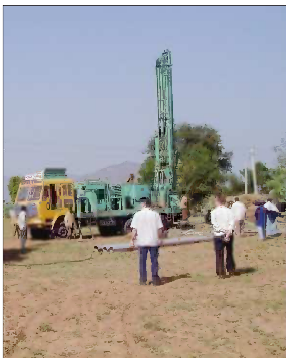
Photo A4.1 Drilling monitoring boreholes in the Satlasana research watershed.
