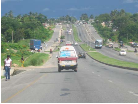
Figure 12 Medium volume urban roads, both divided and undivided, with kerbs and side drains
