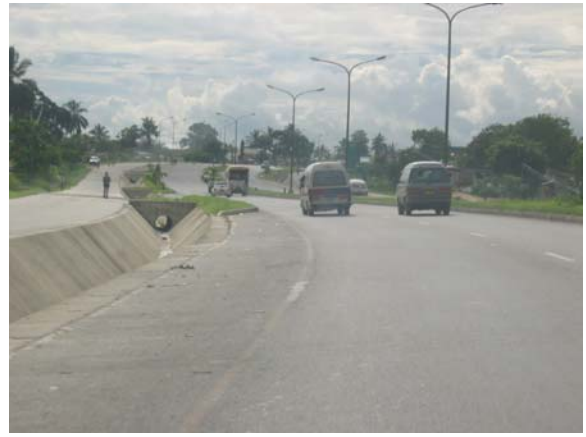
Figure 12 Medium volume urban roads, both divided and undivided, with kerbs and side drains
