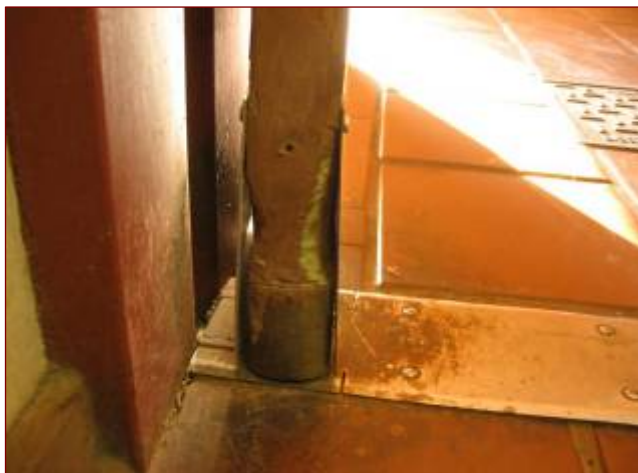
Plate 1.6. Rodent damage to a door in a hospital near Pretoria.
