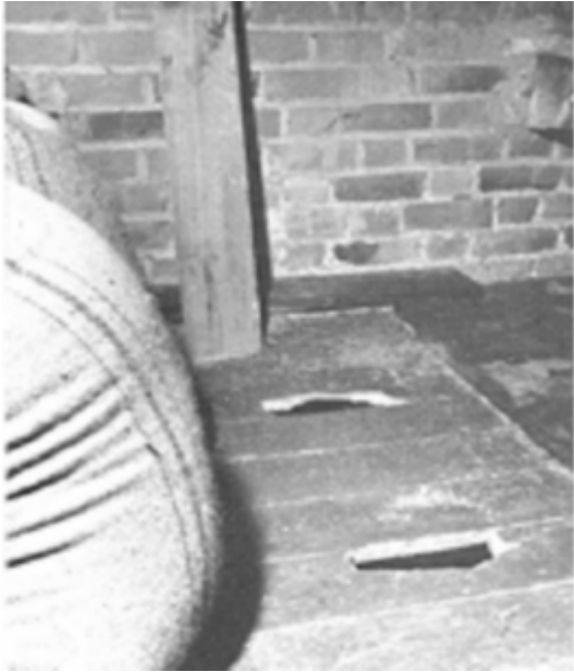
Figure 8.12 Rodent damage to store floor
