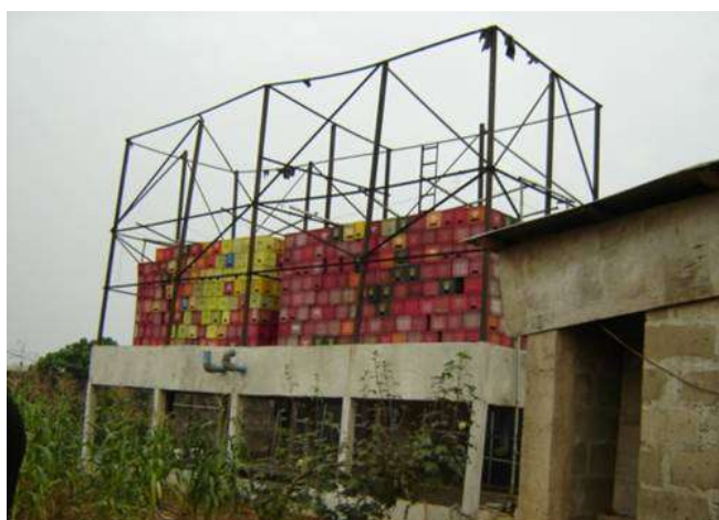
Figure 3: WRS under construction using Crates/lava stones as bio-filter. Lagos state, Nigeria.
