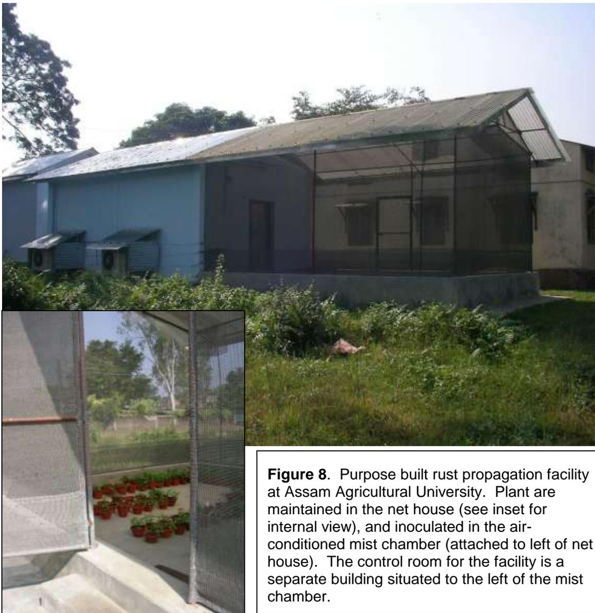
**Figure 8.** Purpose built rust propagation facility at Assam Agricultural University. Plant are maintained in the net house (see inset for internal view), and inoculated in the air-conditioned mist chamber (attached to left of net house). The control room for the facility is a separate building situated to the left of the mist chamber.
