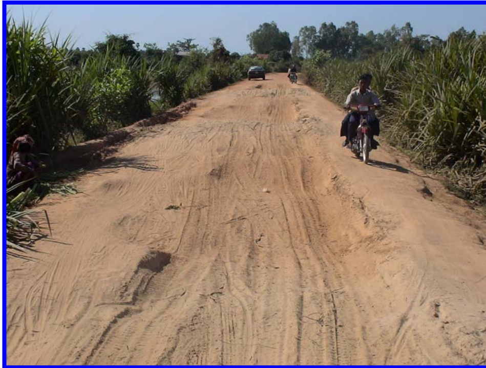
Figure 2.3 – A donor funded project gravel road within 2 years of maintenance cessation (dry season and impassable by motor car!)
