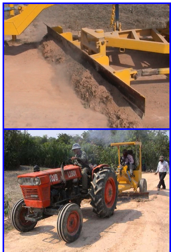
Figure 1.3 - ENGINEERED NATURAL SURFACES: Maintainable using simple locally made equipment
