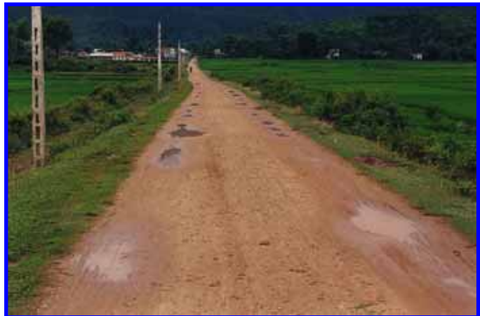
Figure 6.1: Soil shoulders preventing rainfall runoff and effective maintenance grading.
