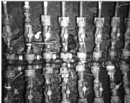
'Durban Tank': Manifold for daily household tank filling IMO Working Group, WSSCC , Kayaga Photos ↑→
