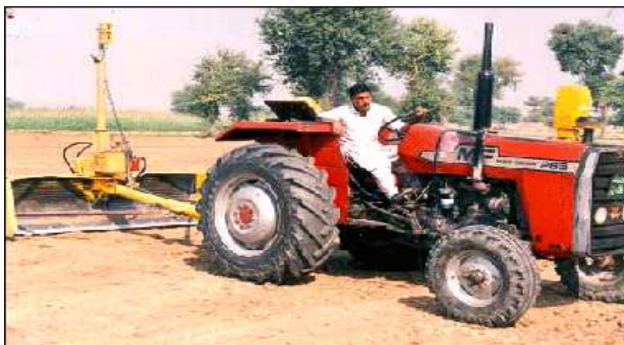
Fig. 4. Laser land levelling in progress
