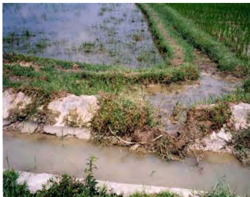
Illegal outlet at SMIP, later replaced by irrigation through field channel from legal outlets
