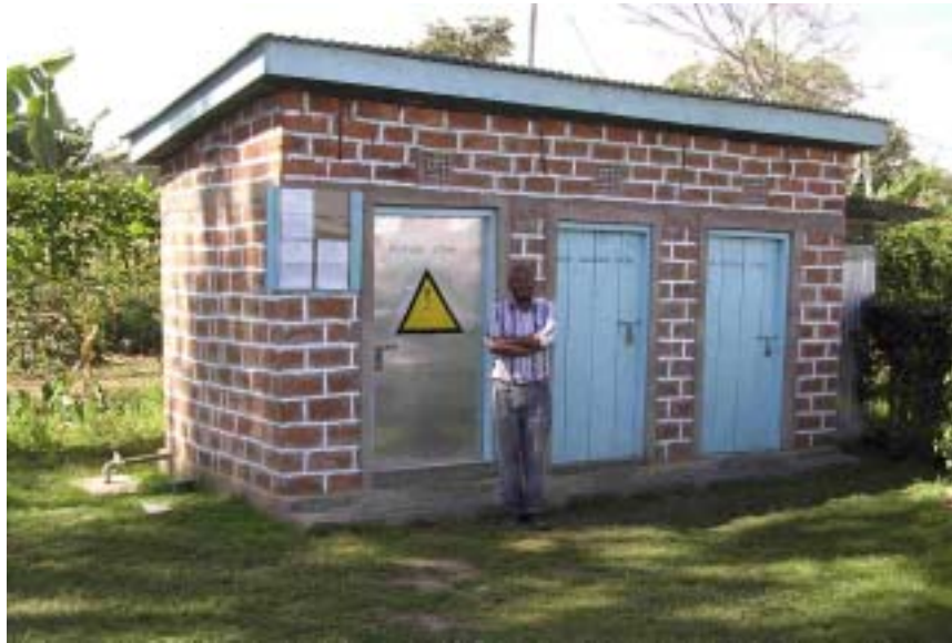
Plate 1: Example of a store for chemicals and equipment, built by a small-scale farmer in Kenya to comply with GlobalGAP
