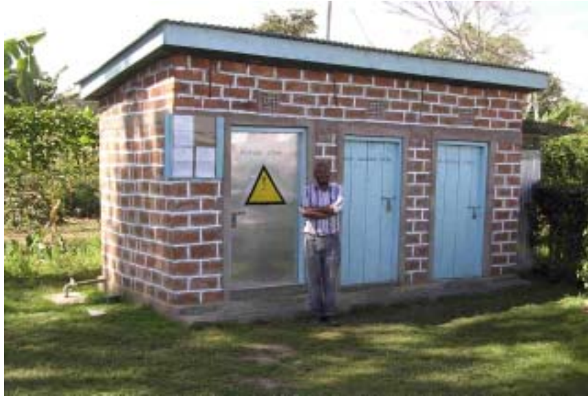
Plate 1: Example of a store for chemicals and equipment, built by a small-scale farmer in Kenya to comply with GlobalGAP
