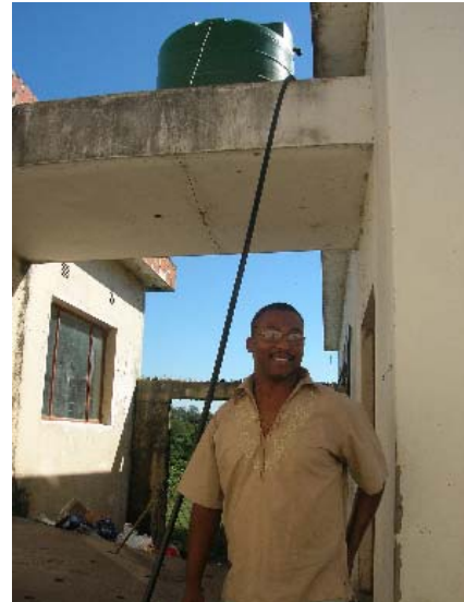
Figure 13.4 An entrepreneur next to the water tank he adapted to fill up automatically when water comes at night
