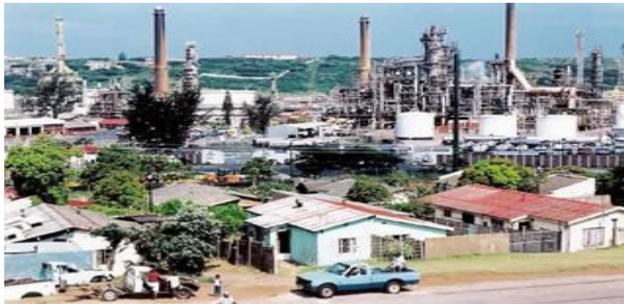
Figure 14.14 Engen Refinery in WentWorth: Shannon Walsh
