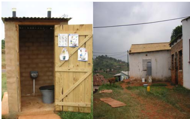
Figure 10.1 Urine Diversion Toilet and 200KL drum, rural and dispersed area in eThekewini Metro
