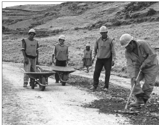
Repairing pot-holes: Micro-enterprises participate in Peru's Rural Road Programme.
