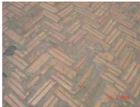
Repaired Mortar Joint
