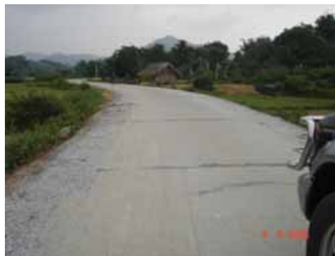
Completed Cement Concrete Pavement
