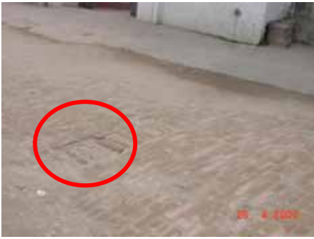
Damaged Bricks
