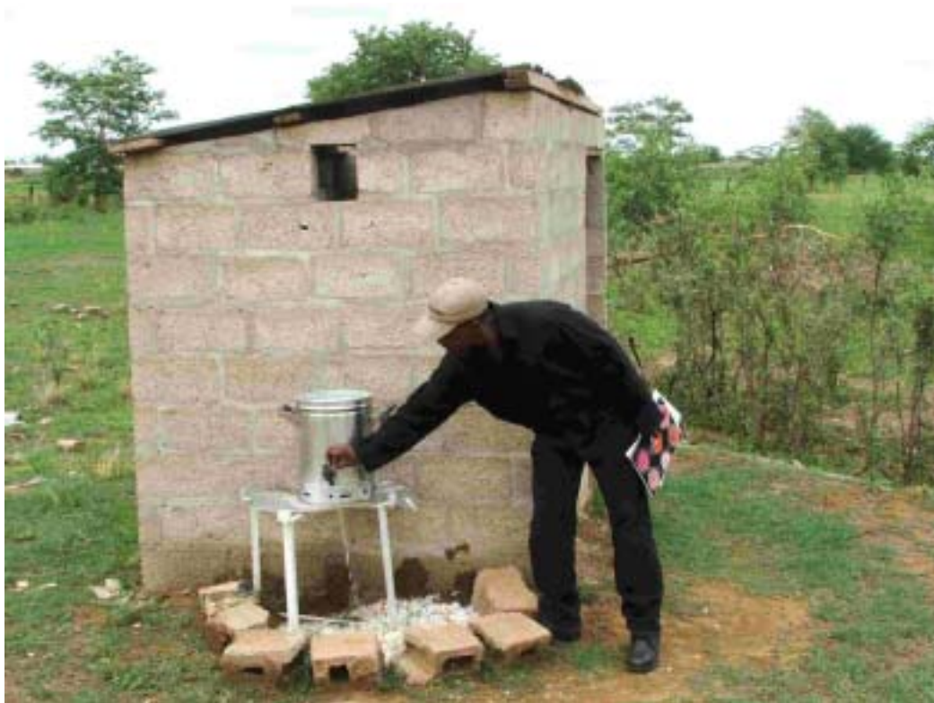
Figure 3. Elaborate field toilet and hand-wash station
