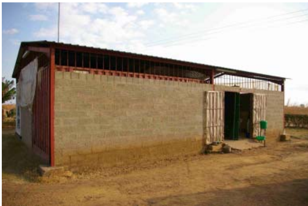
Figure 6. View of the main building at Buteko Depot
