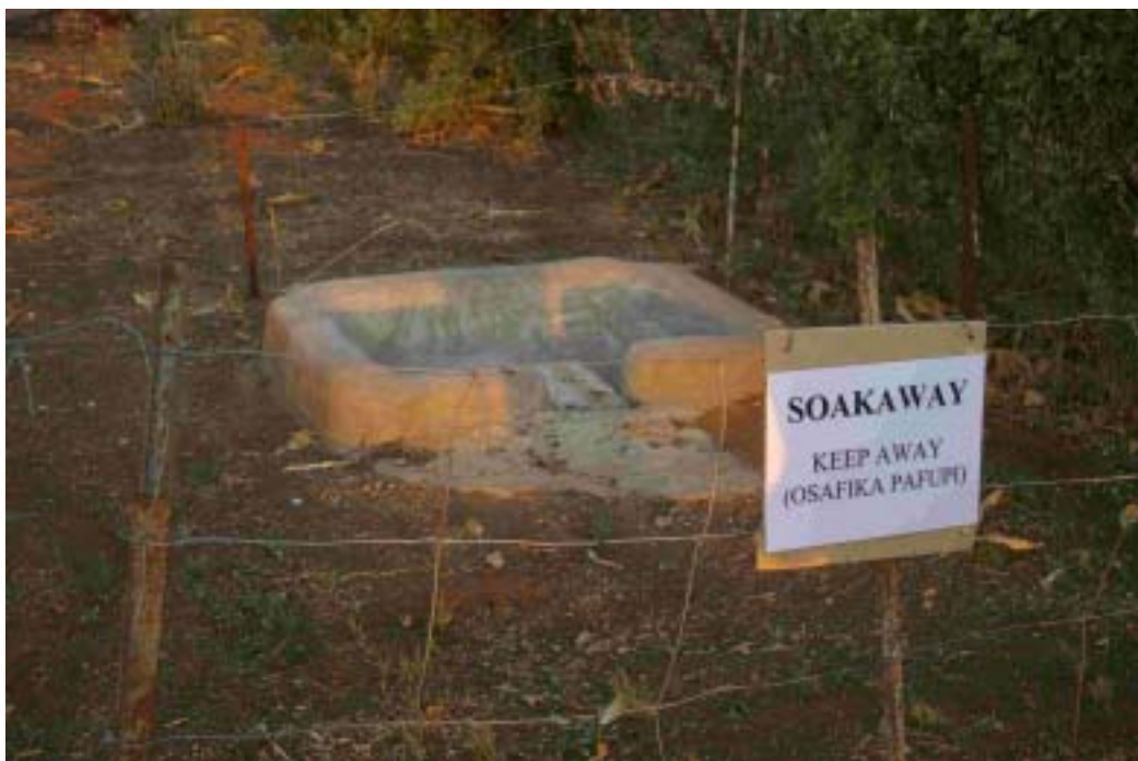
Figure 4. Chemical soak-away for rinsing out CPP sprayers
