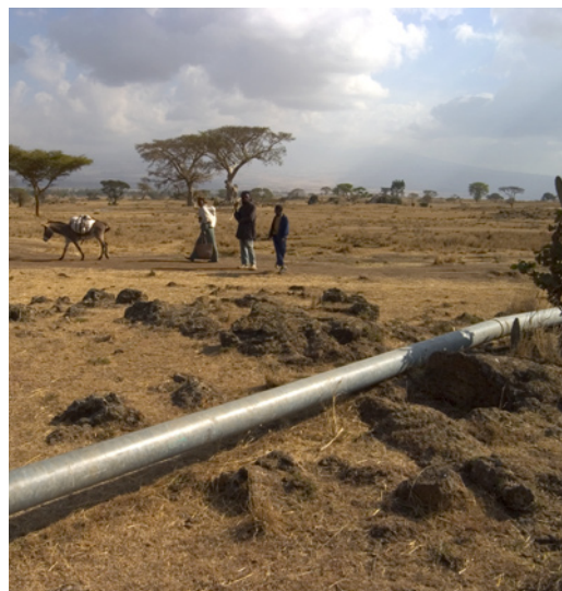
NGO financing paid for this pipeline supplying rural communities
