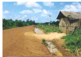
Refill embankment to fill the side drain
