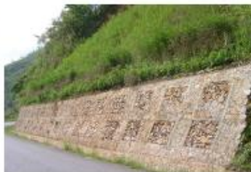
Composite masonry wall
