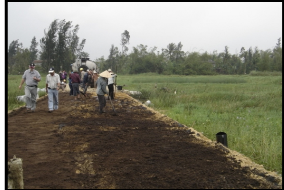
Plate 3 Final hand raking of bitumen emulsion-sand mix
