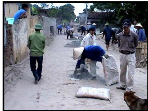
Plate 4 "Spotting" and then breaking bags prior to spreading
