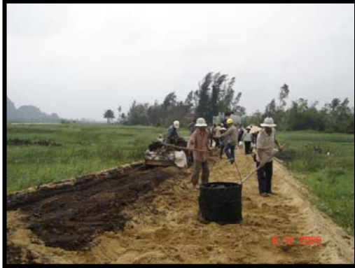
Plate 2 Adding and rotavating bitumen emulsion in short length panels
