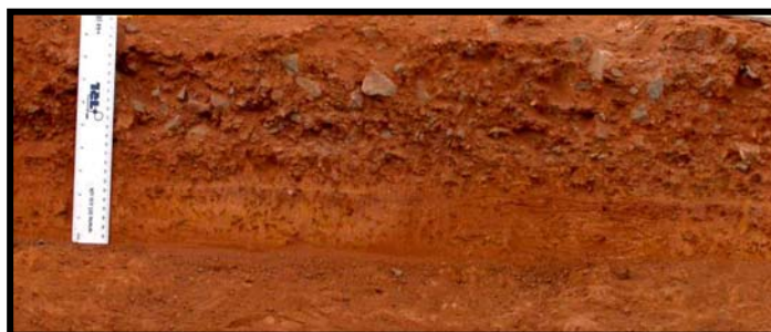
Plate 1 Laterite gravel blended with graded crushed stone as base overlying unblended laterite sub-base
