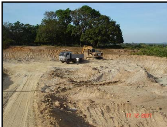
Plate 1 Typical Sand Borrow Pit
