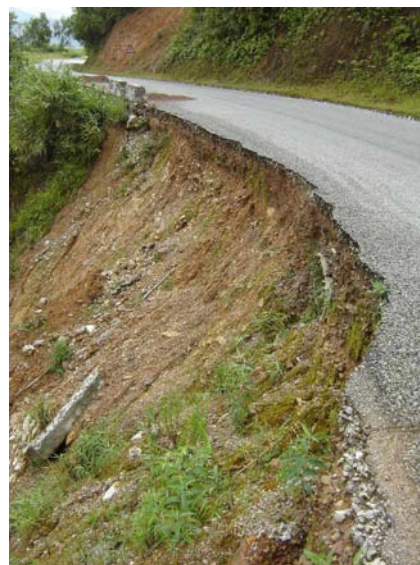
Fig 3. Typical below road failure (assigned Risk No 18)
