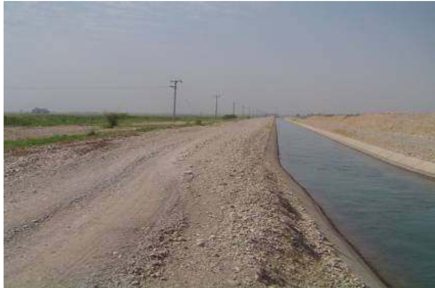
A lined canal receiving water through pumping from Karkheh river
