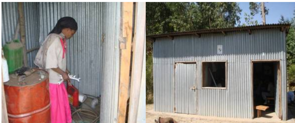
Figure 4.2: Hand tool store and WATSANCo office at Ashoca and Choroqo
