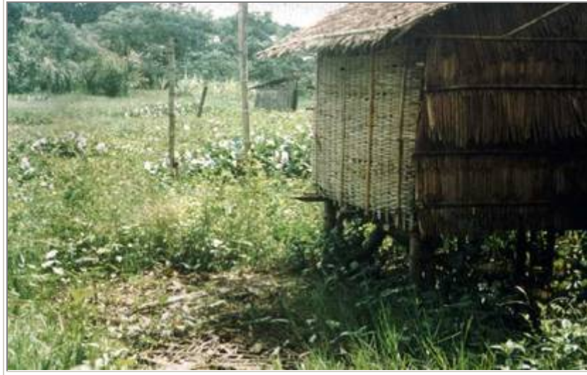
Figure 5: A raised latrine constructed on stilts
