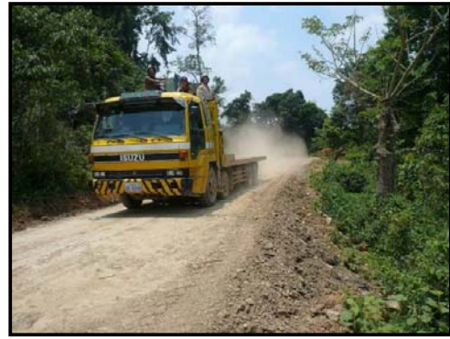
Plate 2. Heavy contractor plant on the Samphan road. One big advantage of the delay in building the spot improvements will be the decreased risk of heavy plant using the trial surfaces
