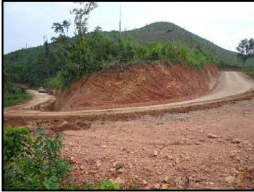
Plate 1. Spot improvement section. Climbing curve at km 2.000
