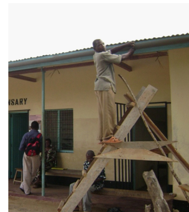
An example of DFF funded maintenance: fixing a gutter to collect rain water
