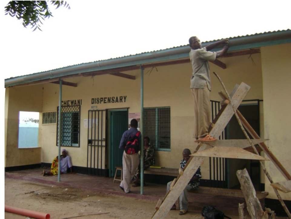
DFF funded maintenance - Fixing gutter for rainwater collection
