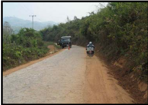
Figure 4.4 Traffic using shoulder rather than rough carriageway
