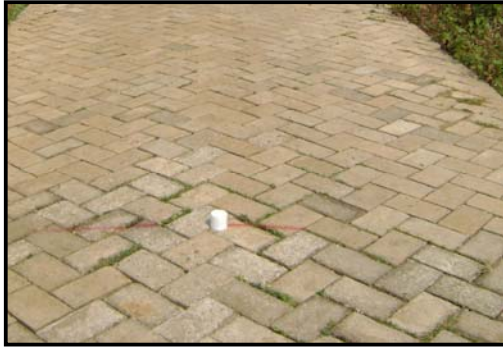
Figure 4.7 Grass growing within joints may loosen blocks
