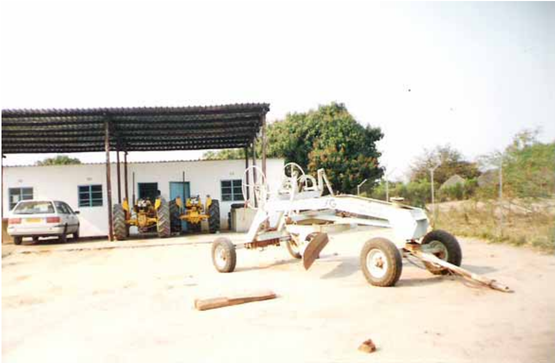
Figure 1: Maintenance Base Camp in Manica
