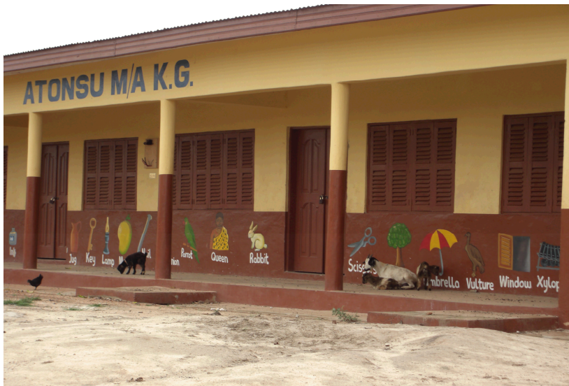
Image 3 – Atonsu Pre-Primary School Wing Constructed in 2007
