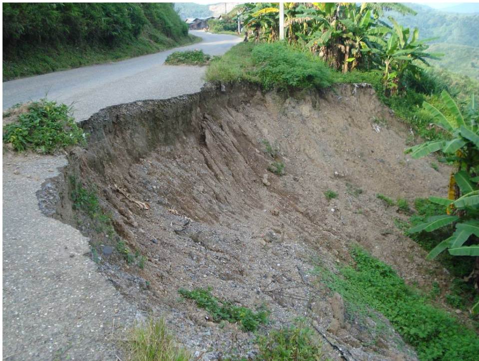
Figure 4 Typical slope failure leading to partial loss of road formation
