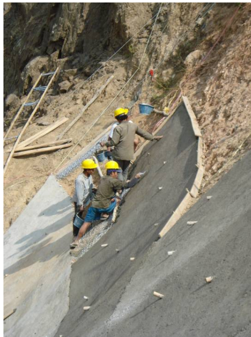
Figure 7 Use of hand-applied reinforced concrete surfacing to stabilise jointed rock masses
