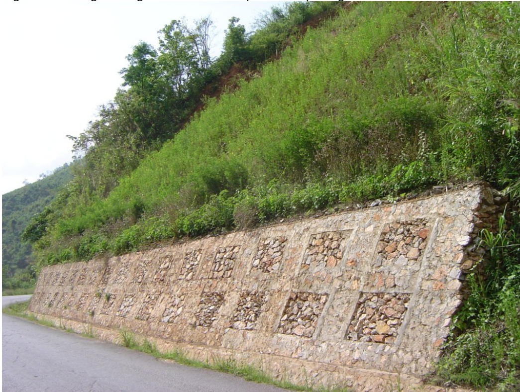
Figure 5 Bio-engineering methods used to protect slopes against shallow failures and erosion
