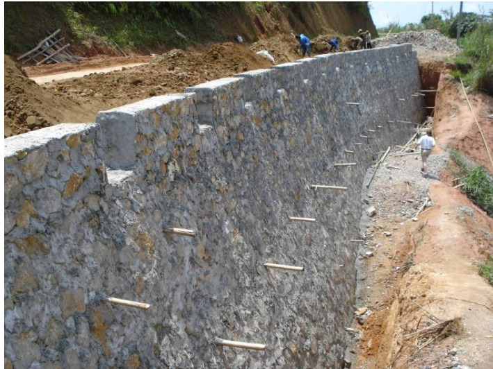
Figure 6 Masonry retaining walls to support the road formation and provide protection from landslides and ground movement on the slopes below
