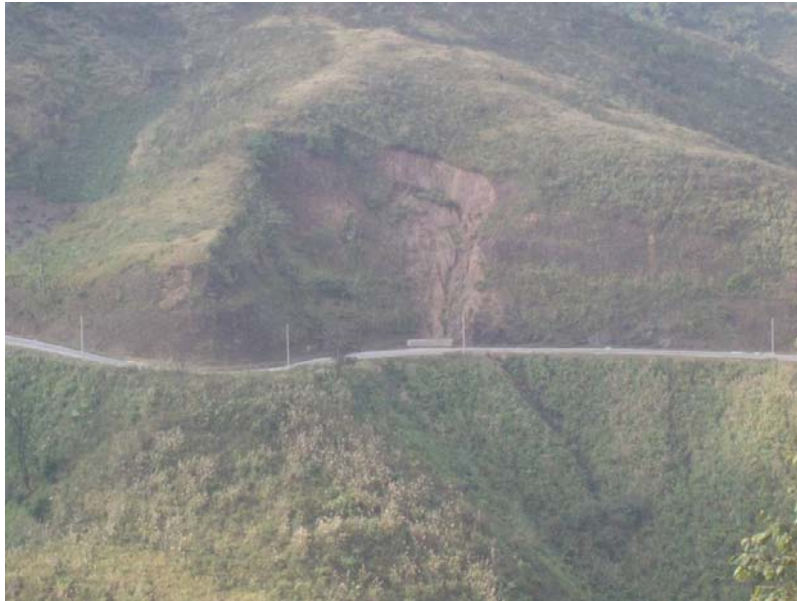
Figure 4 Typical slope failure leading to partial loss of road formation
