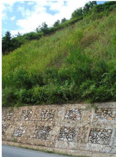
Above-road remedial works using a toe revetment and bio-engineering protection
