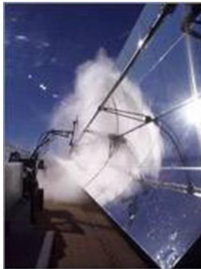
Figure 5: Cleaning trough with water steam (Photo: NREL)
