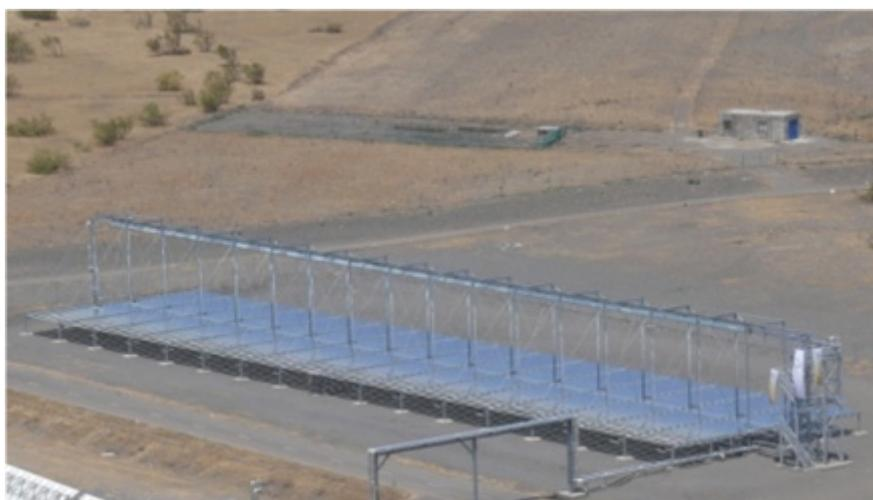
Figure 7: Linear Fresnel solar collector module - demonstration plant
