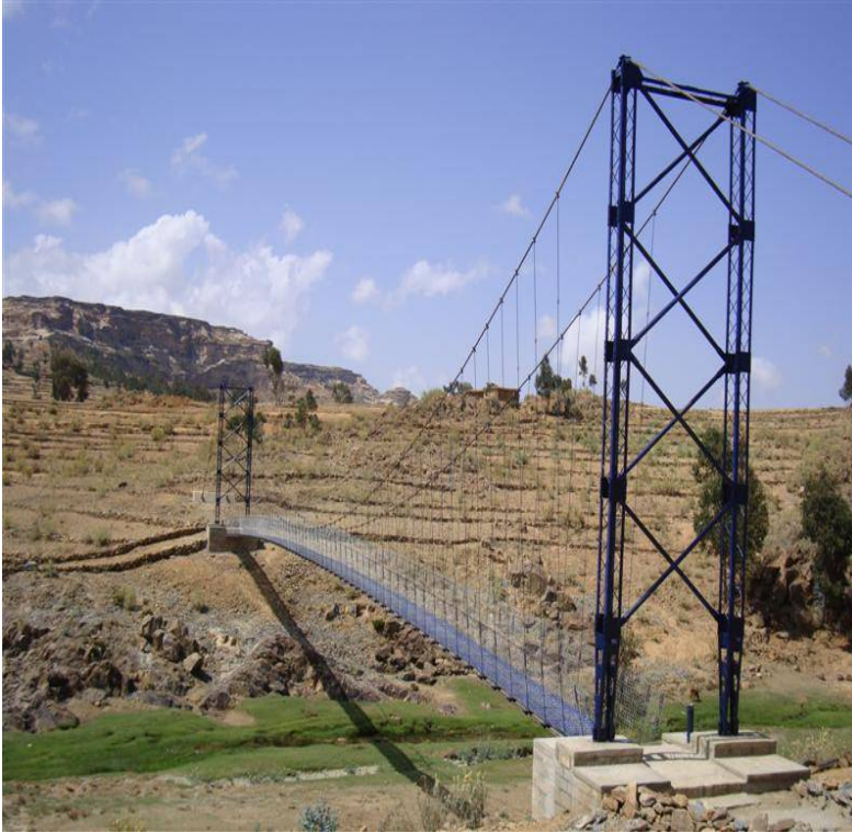
Gerebhidar Trail Bridge, Suspension Type, 73 meters span, Atsbi-Wonberta Woreda, Tigray Region, March 2010
