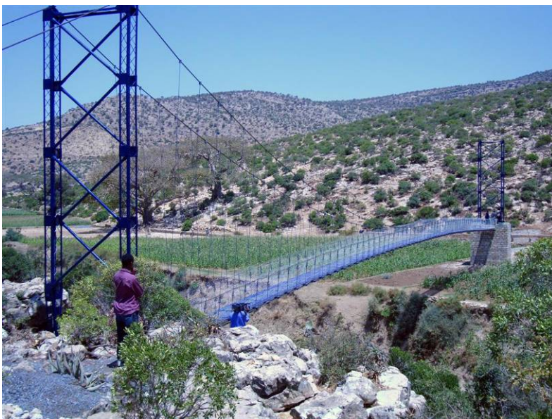
Endamayno Suspension Bridge, Tigray Region, April 2010
