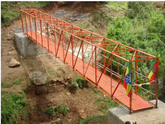
Zemda Steel Truss Bridge, 24 meters span, Yem Special Woreda, SNNPR, April 2010
