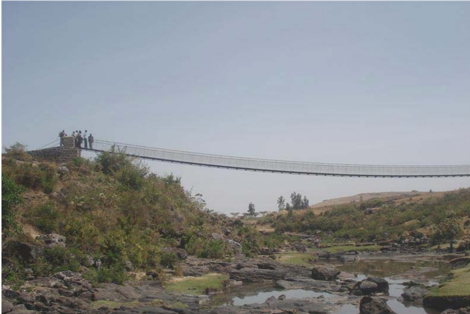
Bale Trail Bridge, Suspended type, 84 meters span, Bale Zone, Oromia Region, 2007
