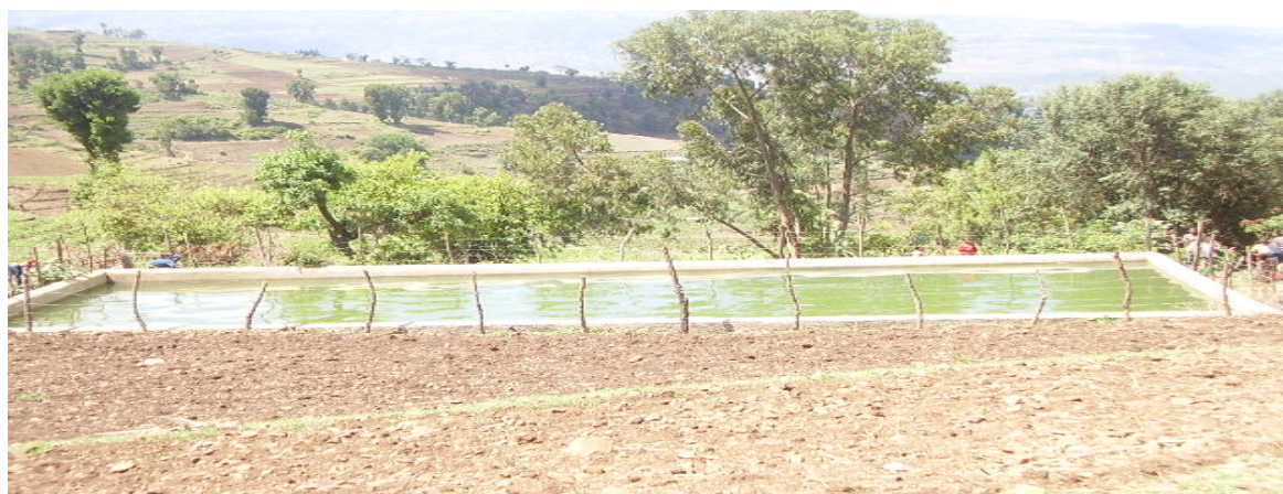
Figure 2.3: View of night storage tank, Ifa Daba
