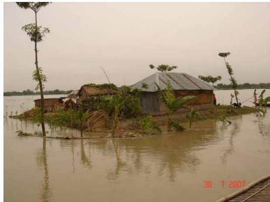
The family is safe and dry on their raised plinth
