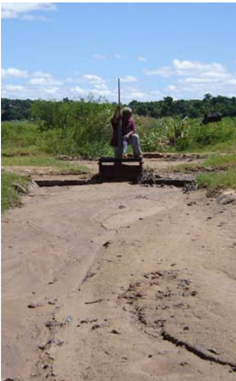
Gap and sand on the main canal called "Karambo" of the check dam of Amboromalandy (Photo : Nosy Alizany, CCAA-Madagascar)
