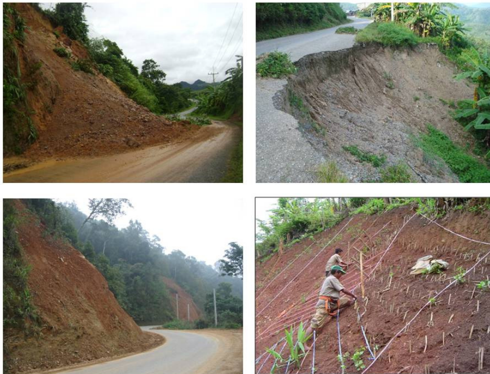
Figure 10 Landslip and remedial works in Laos
