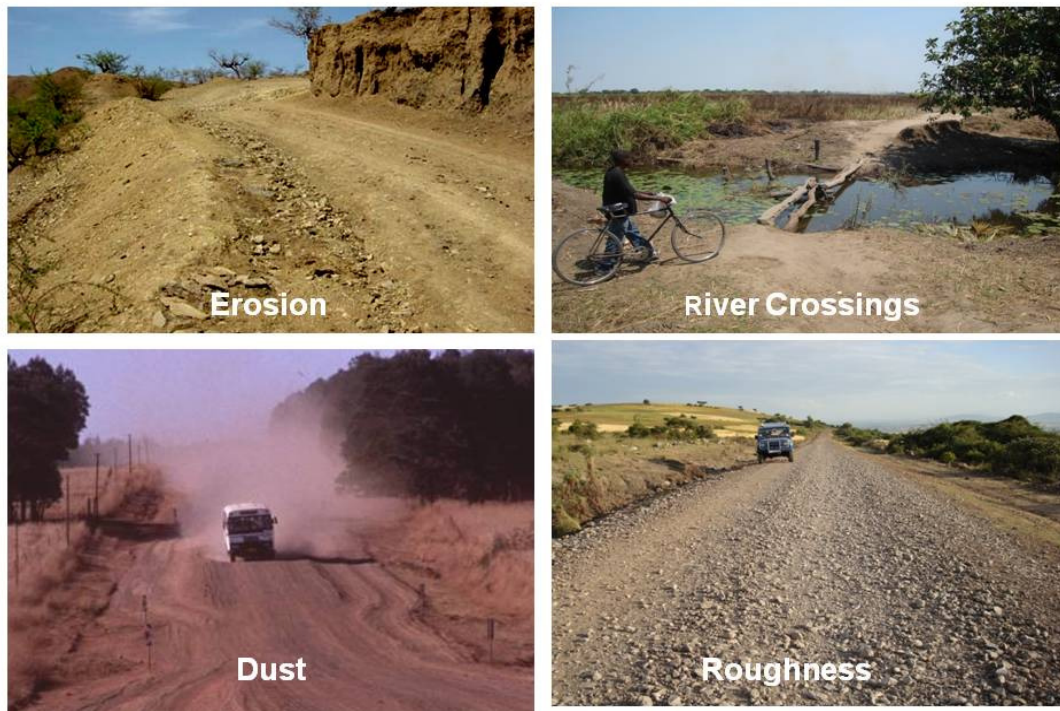
Figure1. Typical problems on gravel road networks
