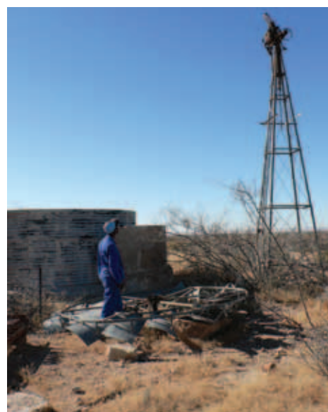
Dilapidated infrastructure on Mara resettlement farm, Maltahöhe District, Hardap Region.
