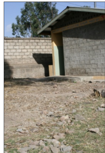
Figure 3 Building material blocks the way to this accessible latrine
