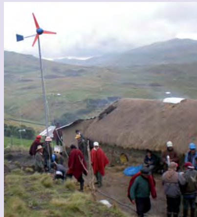
Figure 7.26 – One of 32 100W small wind turbines being installed in 'El Alumbre' in the north Andes of Peru. Three of the individuals shown were trained to install, operate and maintain the systems.
