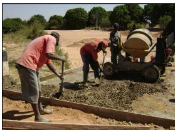
Repair of solid drift on Mphunguzi -Mtita road
