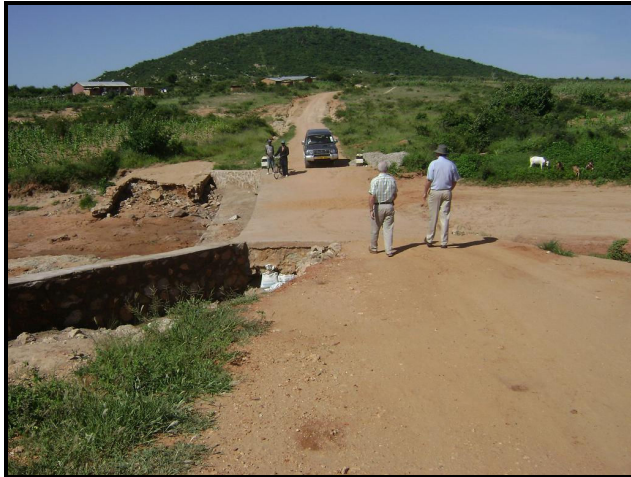
Figure 1: Spot gravelling and culvert construction
