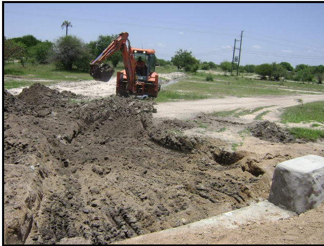
Figure 3: Opening of culvert outlet channel
