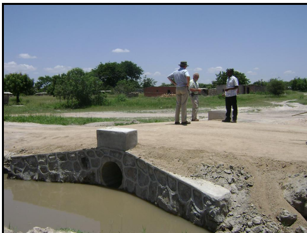
Figure 2: Completed culvert with head and wing walls
