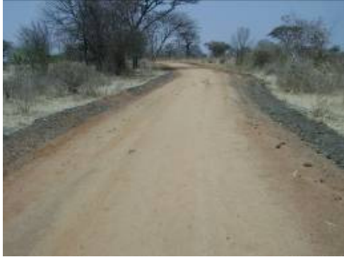
Light grading works done on Mpunguzi - Nkome road
