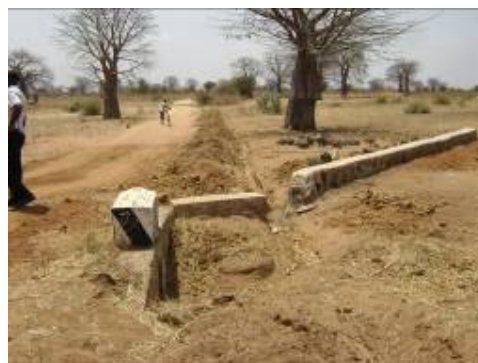
Constructed culvert and extended wing wall on Mundemu – Nguji road
