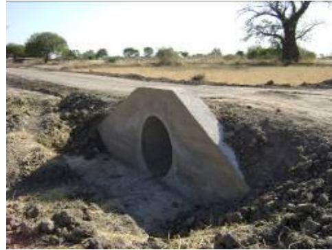
Culvert installation and heavy grading works on Zejele - Nondwa road
