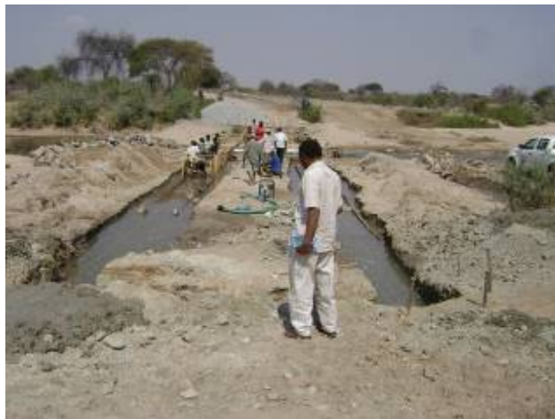
Drift construction works at Chimendele on Bahi – Chimendele road (August 2011)
