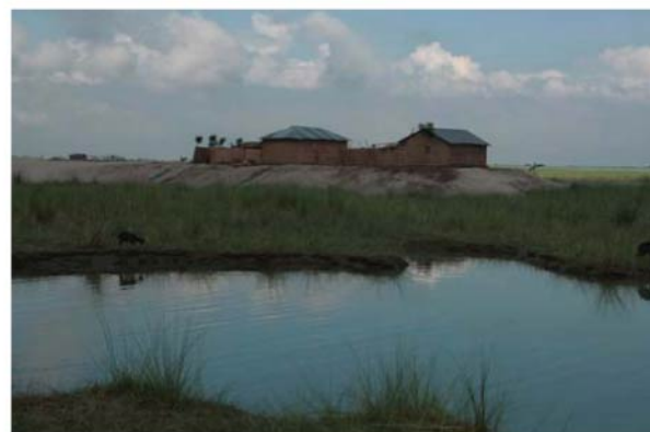
CLP raised plinth
