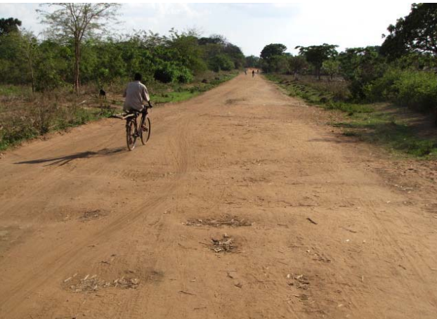
Section of badly rutted and pot holed, gravel section of road in low-lying, poorly drained area
