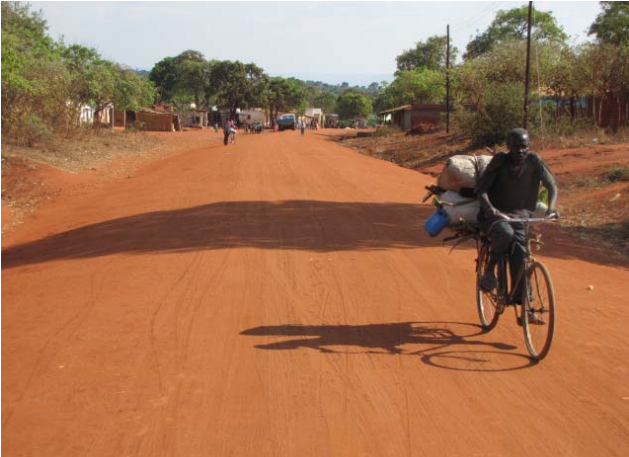
Section of well-formed and drained sandy clay running surface (no gravel wearing course) in good condition near Malingunde
