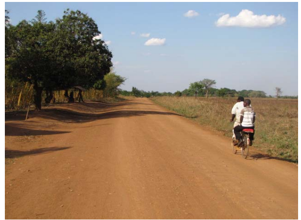
Section of recently graveled section of road in very good condition in reasonably well drained area
