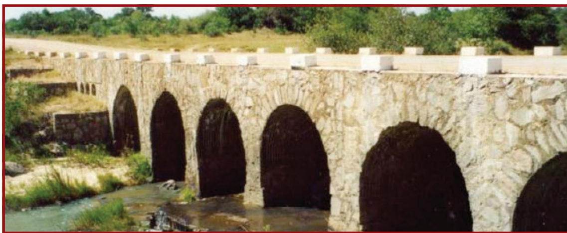
Plate E.4.8: Guide stones on large bore culvert structure
