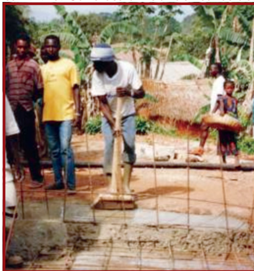
Plate E.7.40: Concrete drift under construction
