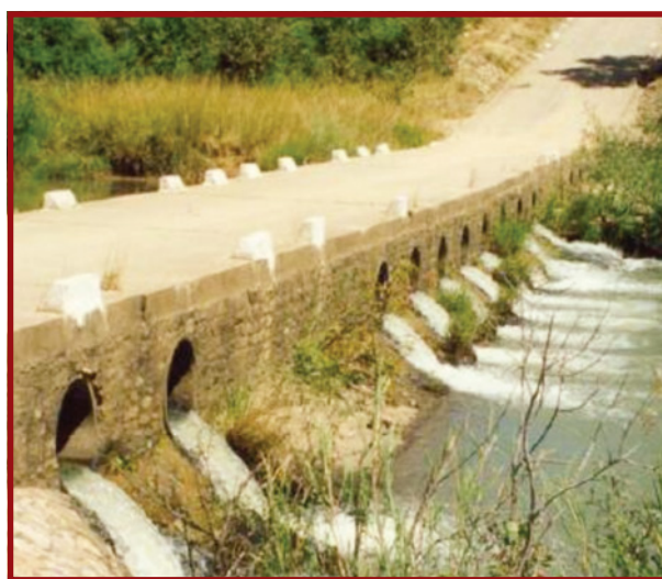
Plate E.4.6: Downstream protection to a vented ford
