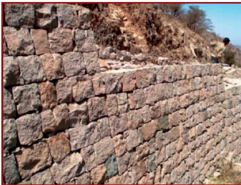
Plate E.7.10: Dressed dry stone wall
