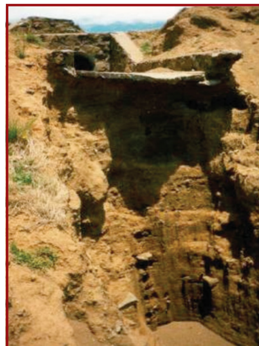
Plate E.8.22: Example of damage due to lack of downstream protection
