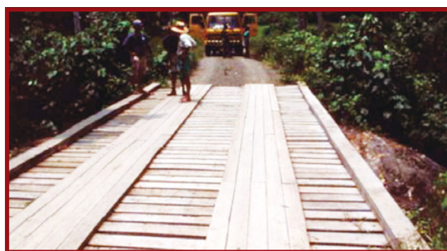
Plate E.7.30: Completed timber deck
