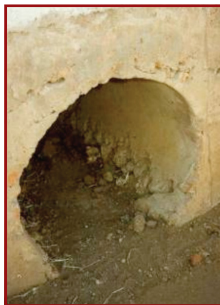
Plate E.8.13: Cast in-situ culvert
