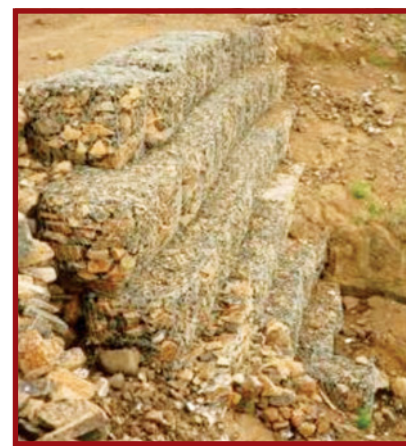
Plate E.7.16: Gabions supporting a road on a steep slope
