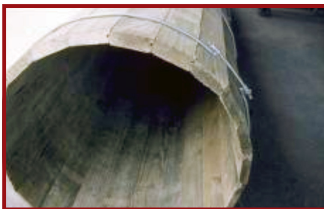
Plate E.8.10: Timber barrel culvert
