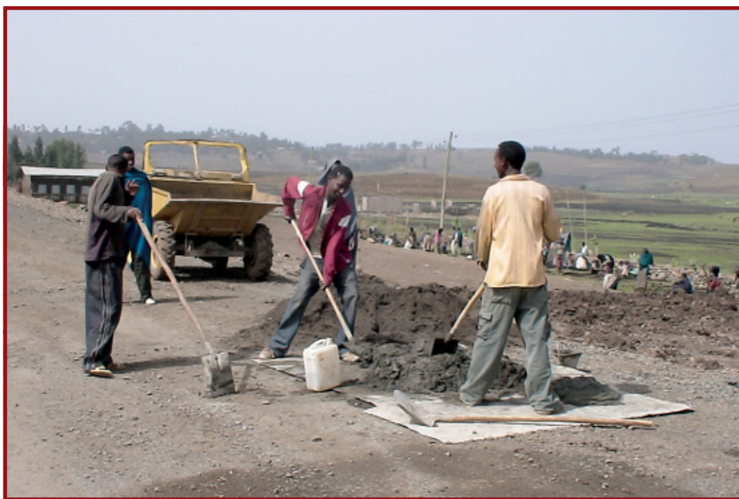
Plate E.9.3: Hand mixing mortar on a clean surface
