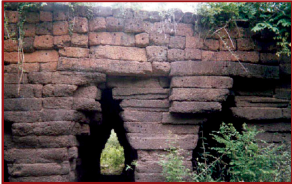
Plate E.7.1: Dry jointed, multiple opening, cantilevered laterite stone culvert approximately 1,000 years old and still in service.
