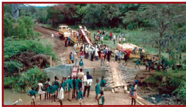
Plate E.7.28: Steel beams being moved into position using labour methods, without the use of cranes; ready for completion with a timber deck
