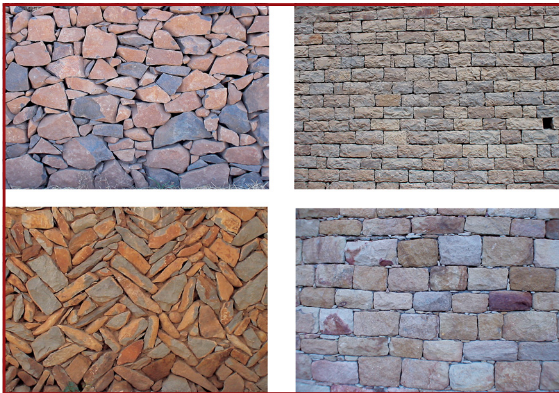
Plate E.7.3: Examples of established Ethiopian techniques of dry stone walling
