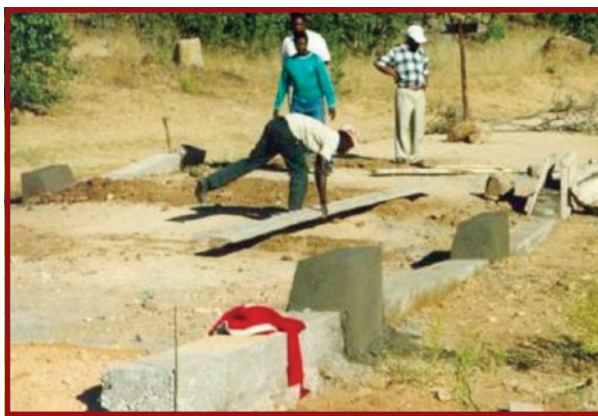
Plate E.8.3: Guide stones at the edge of a drift
