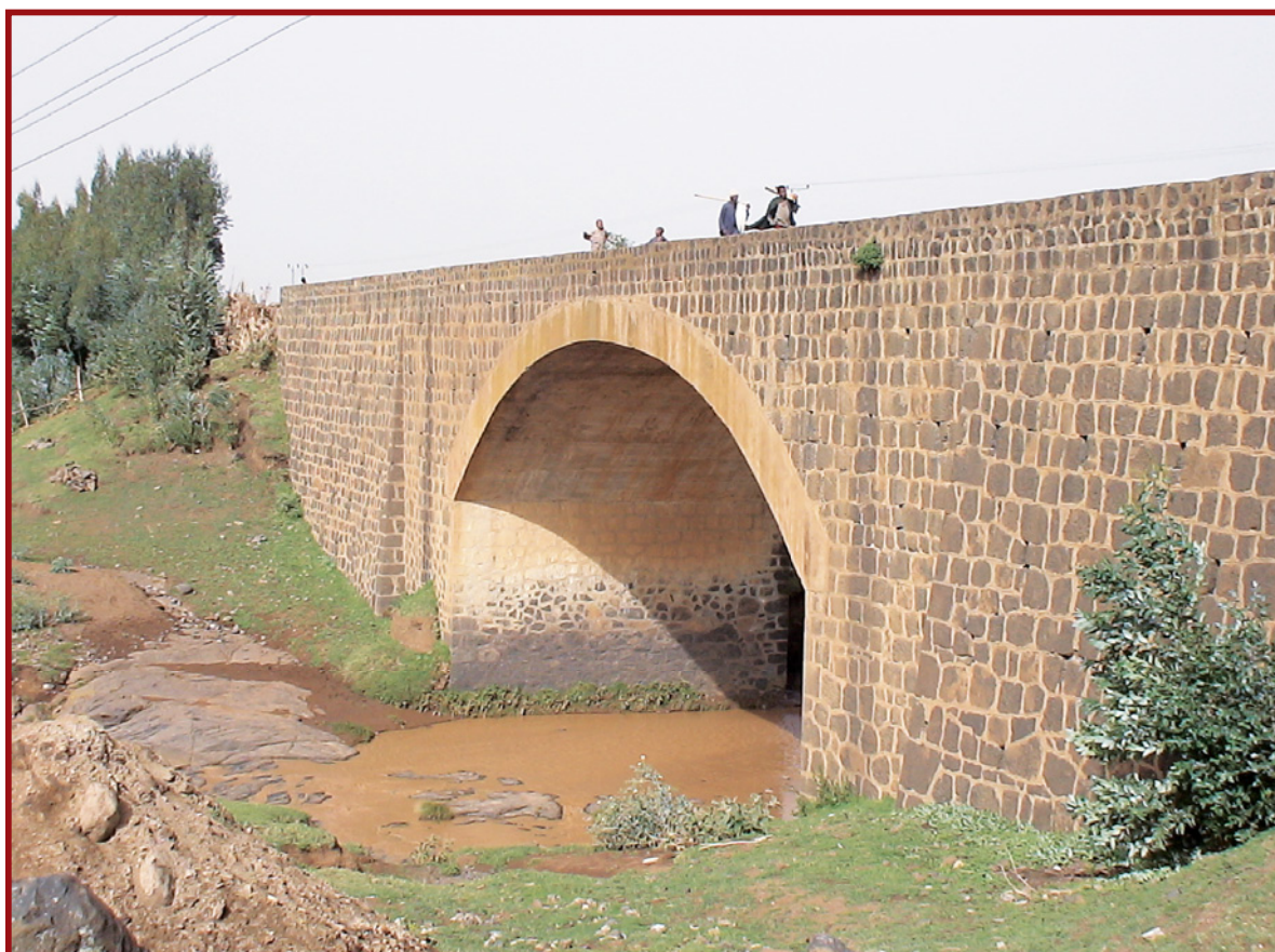
Plate E.1.1: Concrete arch bridge with masonry abutments and spandrels
