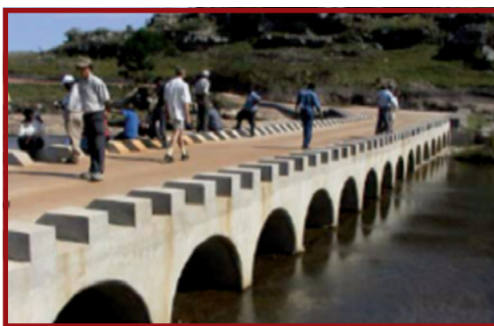
Plate E.8.38: Raised kerbs on a vented causeway allow water to pass over the structure with minimum disturbance, but provide protection from vehicles driving off the structure
