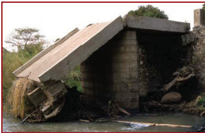
Plate E.8.2: Failure of structure due to a combination of constriction of the watercourse (structure too small), scour and inadequate protection of abutments.
