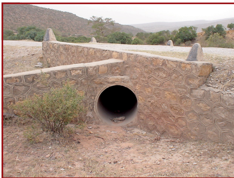
Plate E.8.18: Skew culvert crossing with splay wingwall to prevent water continuing in side drain
