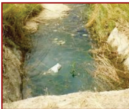
Plate E.8.9: Ponding in outfall channel
