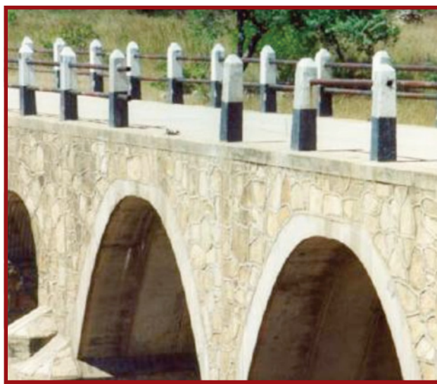
Plate E.3.5: Pedestrian guard rails (in need of repair)
