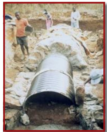
Plate E.7.12: Masonry culvert with steel former to be left insitu after construction
