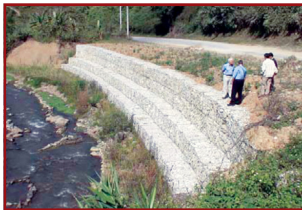
Plate E.7.18: Gabion retaining wall used as river bank protection
