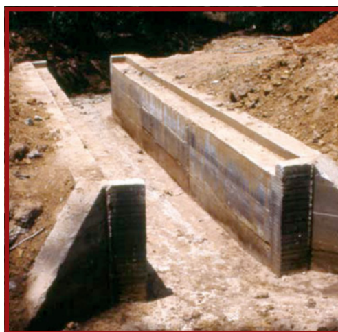
Plate E.7.43: A simple reinforced concrete walled box culvert ready to receive pre-cast top slab units (timber or reinforced concrete)
