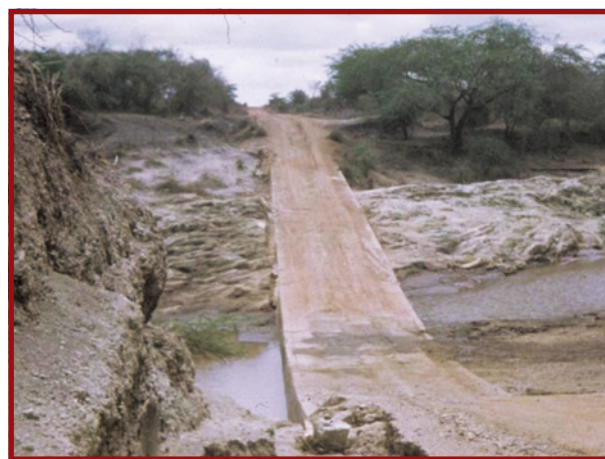
Plate E.4.5: Concrete vented causeway
