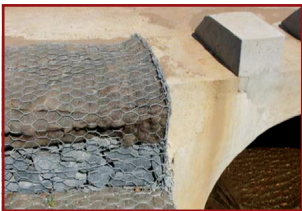
Plate E.7.19: Natural fibre matting inserted in gabion protection works to encourage rapid growth of vegetation cover
