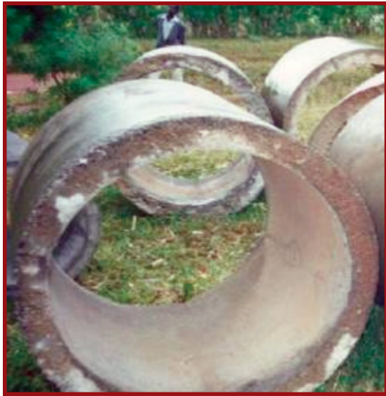
Plate E.8.15: Precast concrete culvert ring
