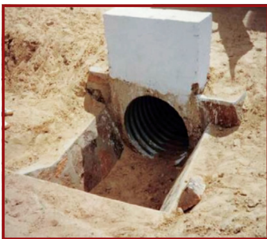
Plate E.5.5 and Figure E.5.4: Culvert drop inlets
