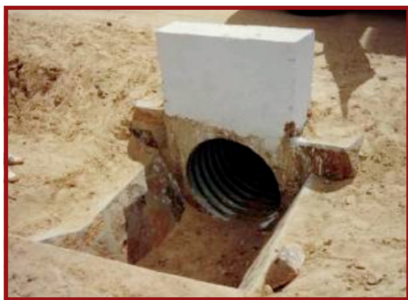
Plate E.8.17: Drop inlet on stream culvert
