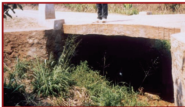
Plate E.10.3: Box culvert partially blocked by vegetation
