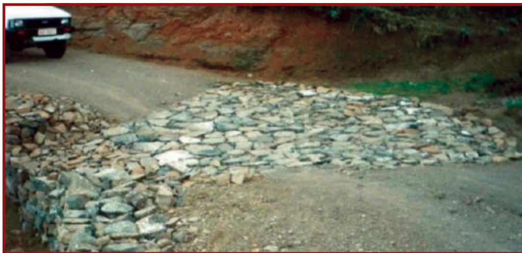
Plate E.8.5: Hand pitched stone drift
