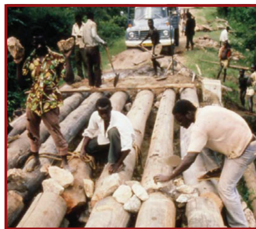
Plate E.7.33: Timber poles as deck beams of a twin span bridge
