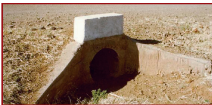
Plate E.3.3: Culvert head stone outside main running lanes
