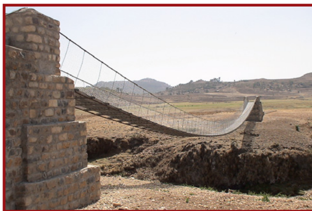
Plate E.1.3: Steel cable pedestrian bridge
