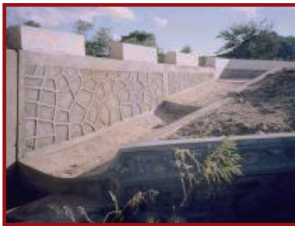
Plate E.8.21: Masonry side drains at the edge of an approach way
