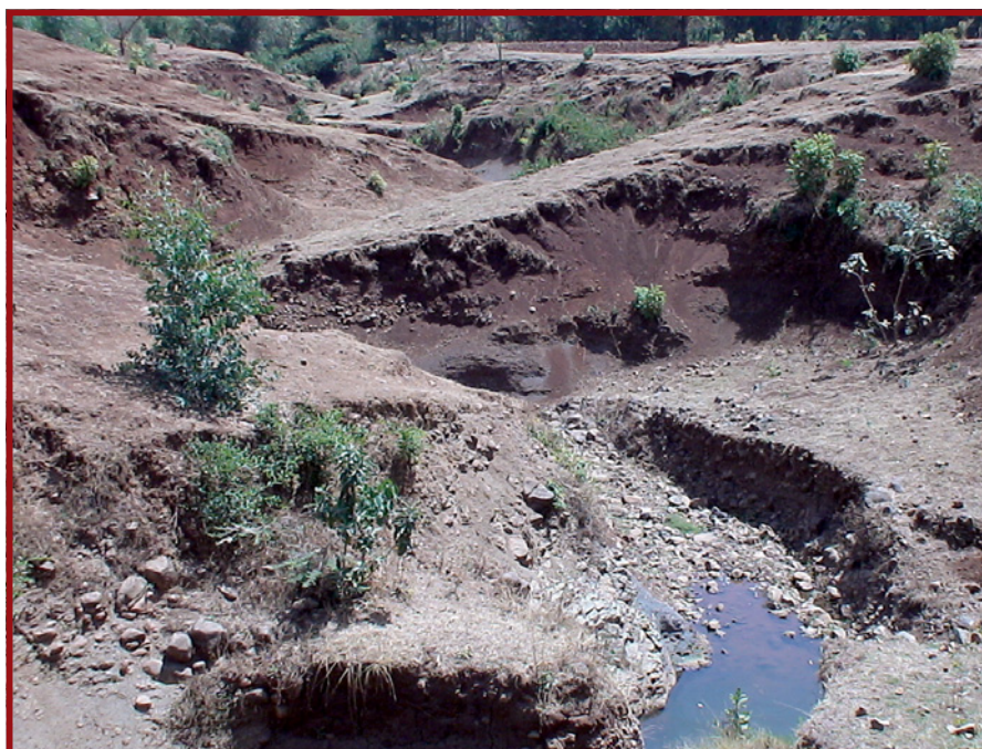
Plate E.8.24: Serious erosion downstream from the same culvert due to concentration of flow and lack of appropriate protection measures
