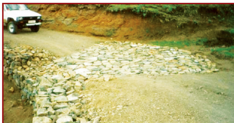
Plate E.4.2: A basic hand packed stone drift
