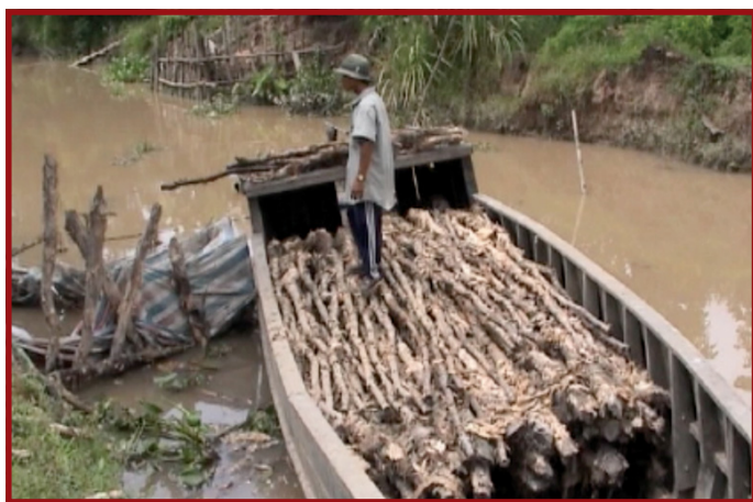
Plate E.7.32: Timber poles for piles (not covered by this Manual) for a concrete box culvert in very soft ground
