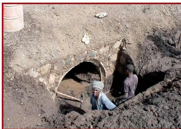
Plate E.10.4: Cleaning the drop inlet and barrel of a large bore culvert
