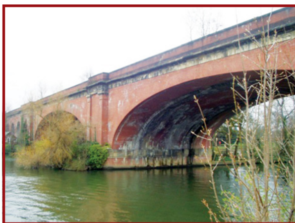
Plate E.7.22: Fired clay brick is a very versatile material. This elliptical brick arch bridge over the River Thames at Maidenhead, UK was constructed in 1838 and has two main spans of 38 metres. It is still in use today (designer: Isambard Kingdom Brunel) photograph by Jon Combe
