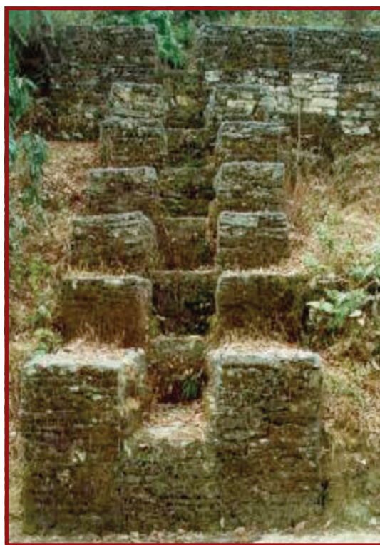
Plate E.8.28: Gabion basket step waterfall
