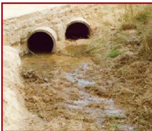
Plate E.5.3: Ponding at culvert outlet
