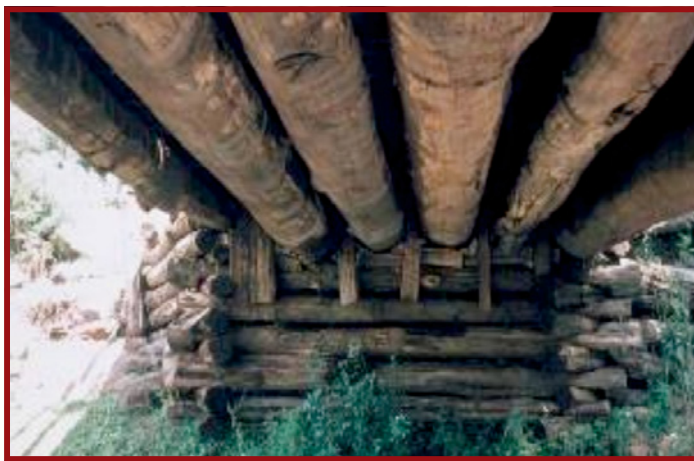
Plate E.7.35: Log abutments & deck
