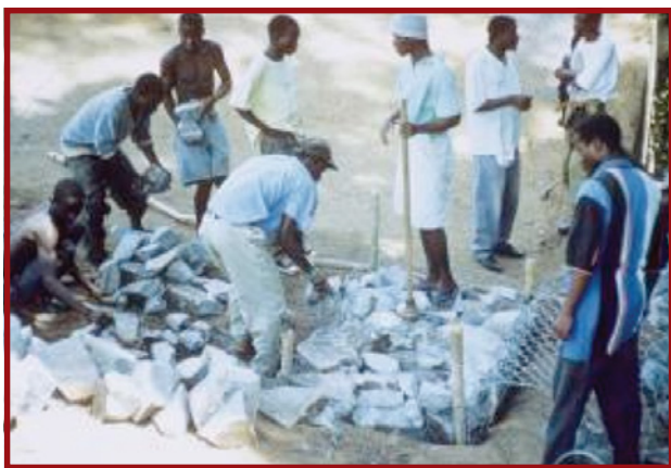
Plate E.7.17: Filling gabion baskets
