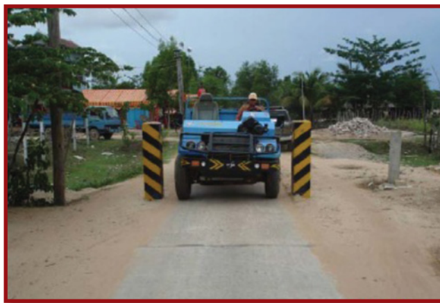
Plate E.3.2: Robust width restrictions can be used in some instances to restrict heavy vehicles
