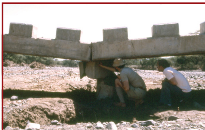
Plate E.5.1: Collapse due to settlement
