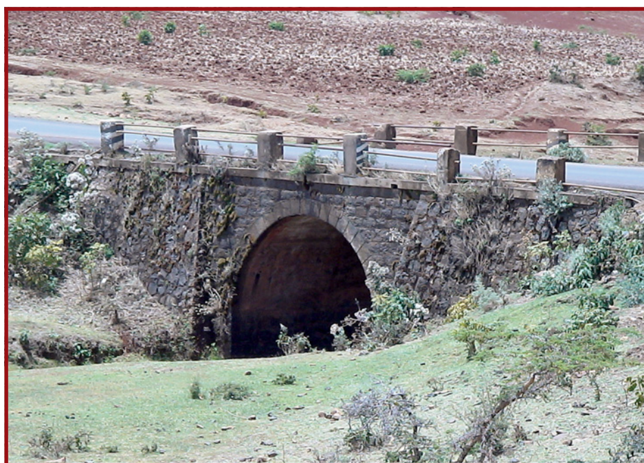
Plate E.8.30: Semi-circular Arch bridge
