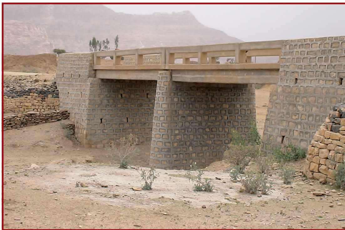
Plate E.8.31: Two span concrete deck bridge with masonry pier and abutments
