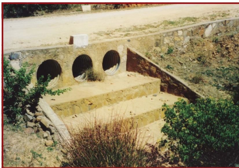
Plate E.4.3: A three barrel corrugated steel culvert with stepped outfall apron
