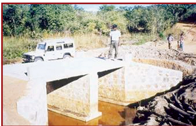
Plate E.8.32: Reinforced concrete deck on masonry abutments and pier
