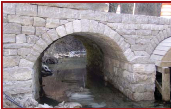
Plates E.7.13-15: Dry stone masonry culvert extension works - Dry stone Conservancy, USA
