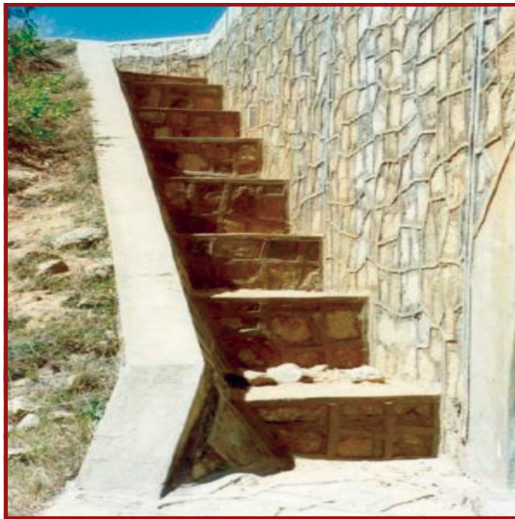
Plate E.8.20: Wingwall cascade
