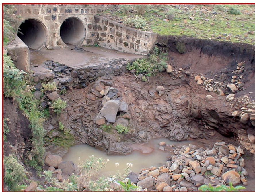
Plate E.8.26: Severe erosion downstream of a cross culvert due to inadequate protection measures
