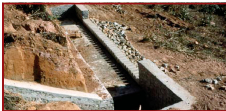
Plate E.7.42: Flow spreader structure at the outlet of a mitre drain on a steep fragile slope. Bio-engineering planting should be established downhill of such structures
