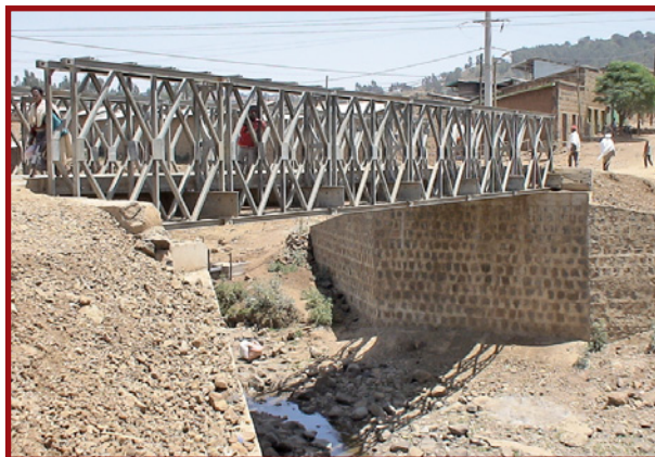
Plate E.1.2: Modular steel panel bridge
