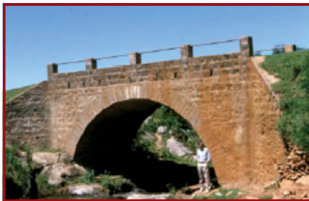
Plate E.8.34: Completed masonry arch bridge with splayed wing walls on hard rock foundations
