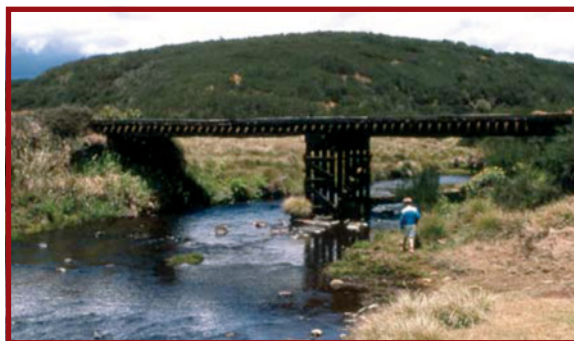
Plate E.7.31: Timber bridge deck, pier and abutments
