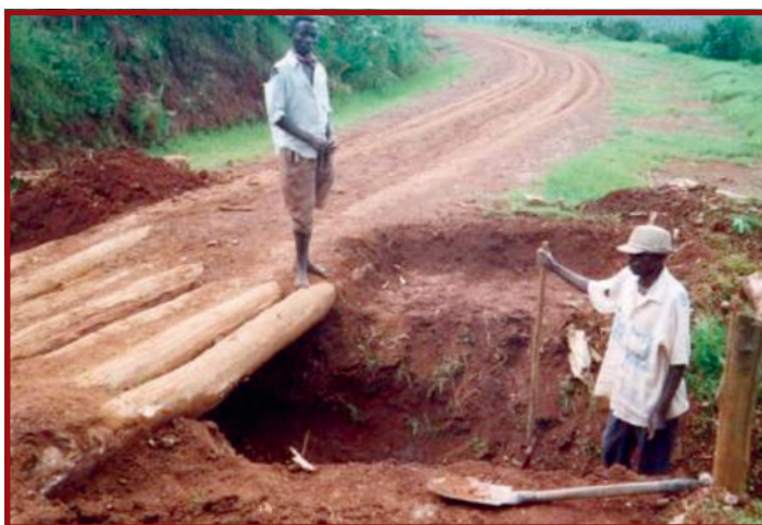
Plate E.8.11: Timber pole culvert during reconstruction
