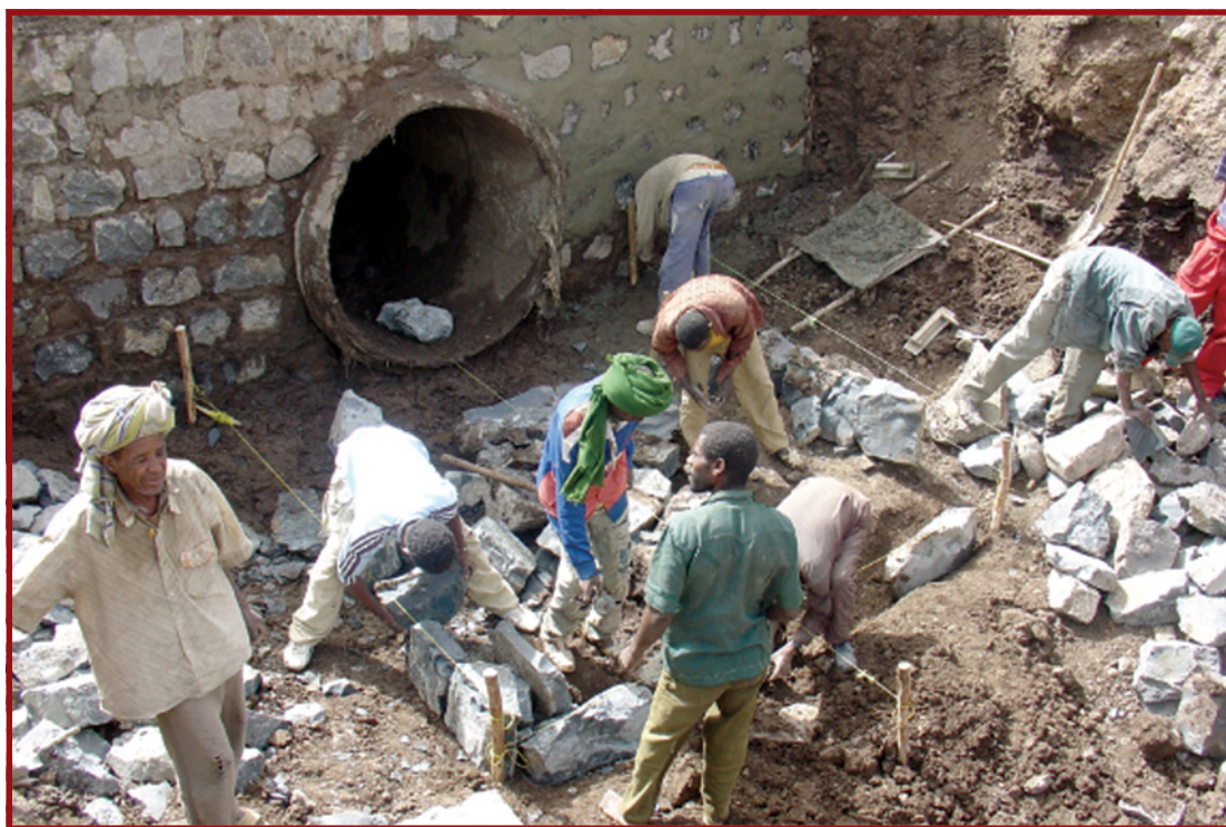
Plate E.9.1: Construction of culvert inlet apron with guide pegs and strings
