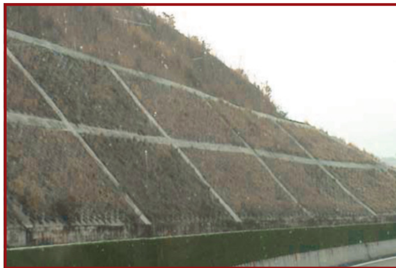
Plate E.7.11: Hybrid retaining wall
