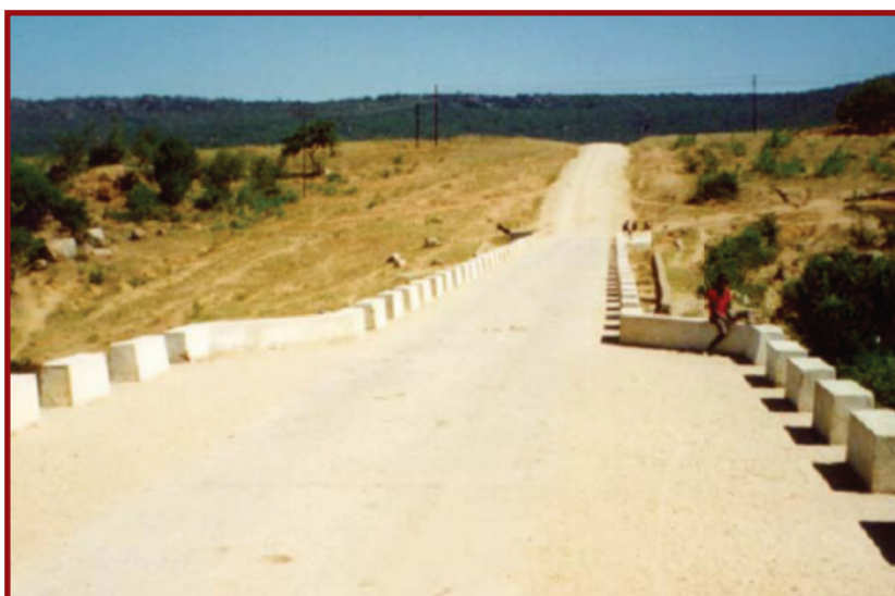
Plate E.3.4: Guide stones narrowing road width
