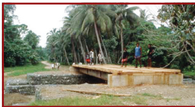
Plate E.7.29: Timber deck on recycled steel beams
