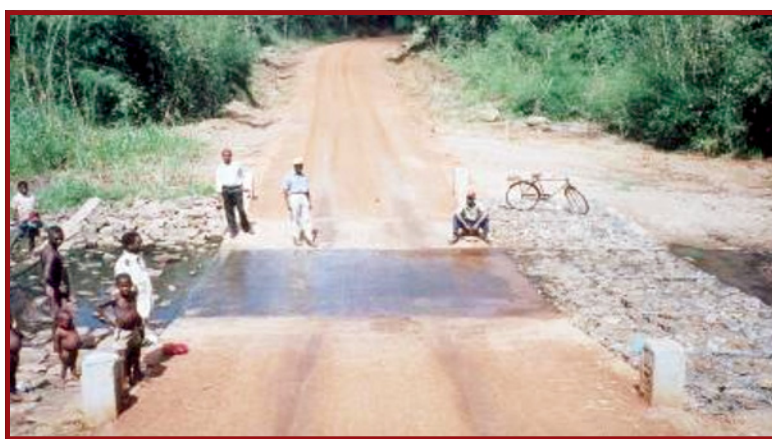
Plate E.8.4: Concrete slab drift
