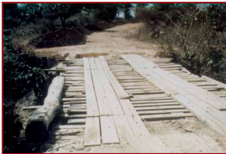
Plate E.8.35: Timber deck with floor planking and edge beams in need of repair
