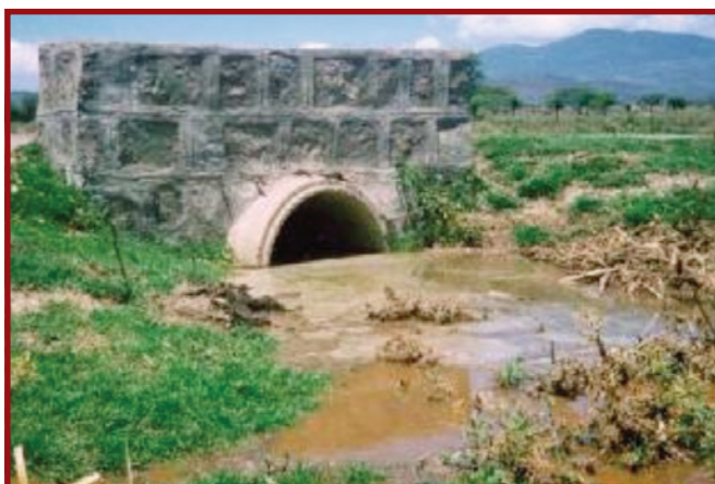
Plate E.8.8: Ponding at culvert outfall
