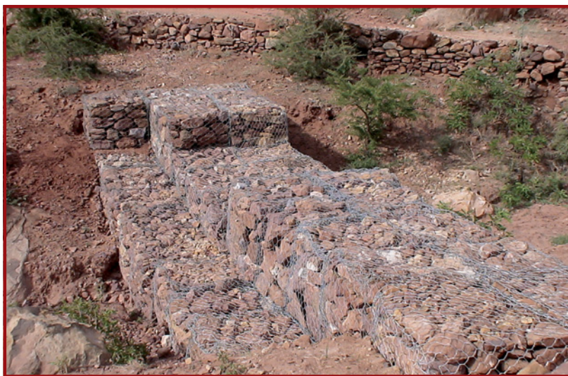
Plate E.8.27: Gabion erosion control structure downstream of a culvert
