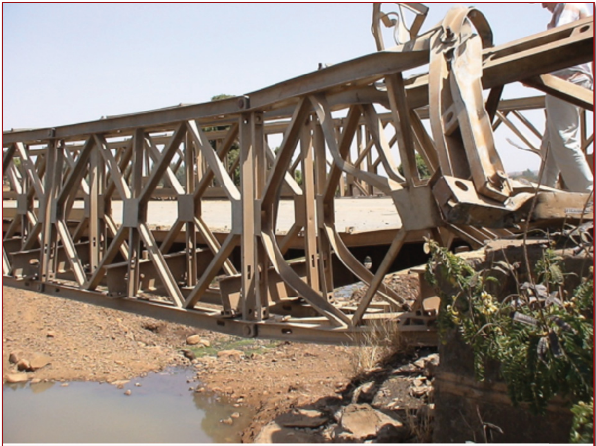
Plate E.10.5: Serious vehicle impact damage to steel panel bridge
