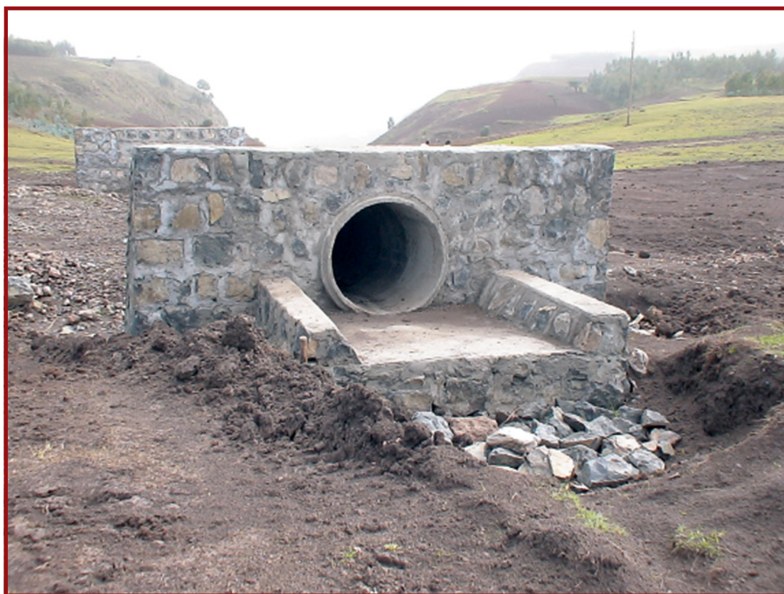
Plate E.9.2: Completed culvert inlet apron
