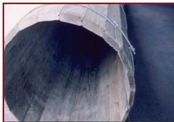
Plate E.9.4: Timber stave culvert
