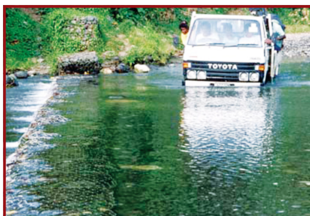
Plate E.7.21: Gabion river crossing
