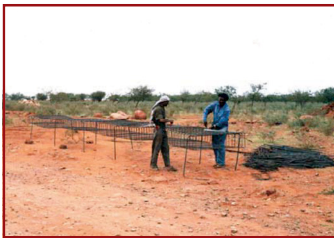
Plate E.7.38: Steel reinforcement cage being assembled
