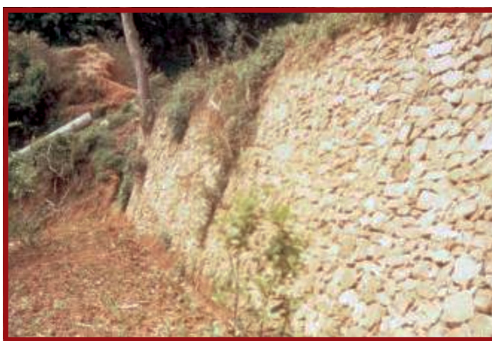
Plate E.7.9: Dry stone wall supporting embankment
