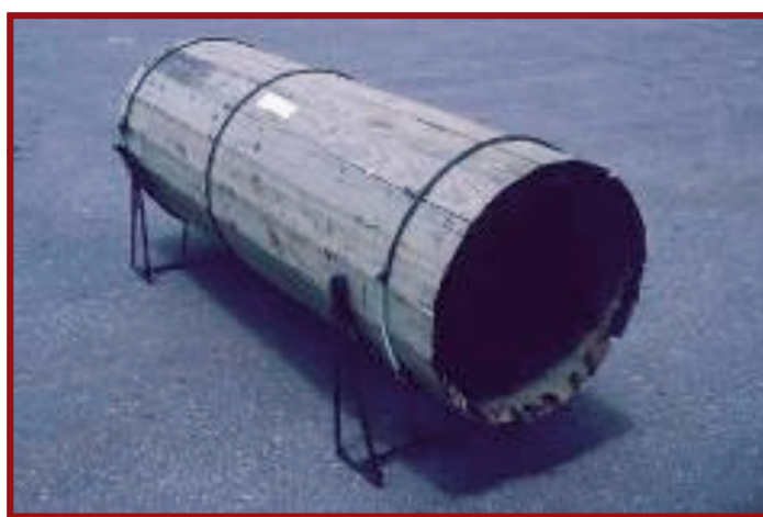
Plate E.7.36: Treated timber culvert
