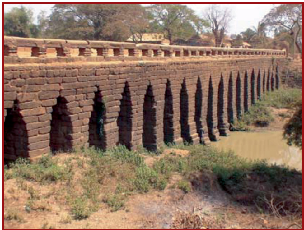
Plate E.7.2: Dry jointed, laterite, stone viaduct, approximately 1,000 years old, still in service on a main road.
