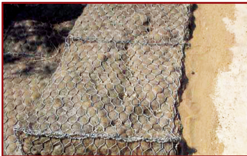
Plate E.8.7: Natural fibre matting inserted in the top and face of the gabion
