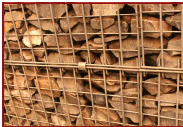
Plate E.7.20: Steel mesh gabions
