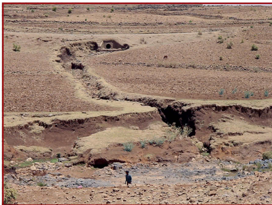
Plate E.8.25: Severe erosion downstream of a relief culvert due to inadequate protection measures
