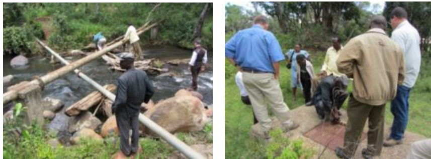
FIGURE 2. LOCATION OF BULK WATER ABSTRACTION AND MANUAL METERS ON THE BURGURET RIVER
