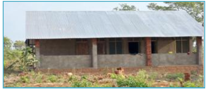
Dispensary under construction in Kiswago village as part of the PHSDP
