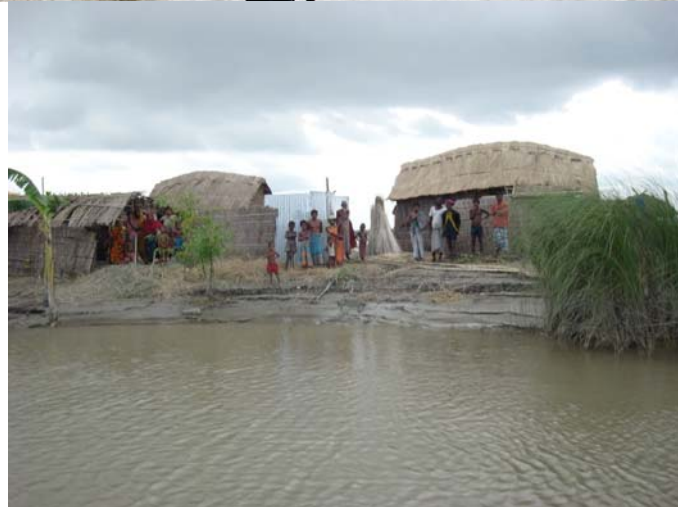
A cluster of homesteads on a CLP raised plinth
